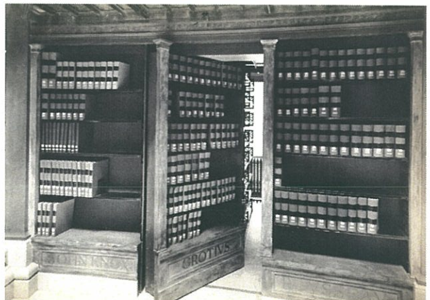
fig. II-17 Gould Memorial Library wall of bookshelves with pivoting door to stacks, Courtesy of New York University Archive-Bobst Library
