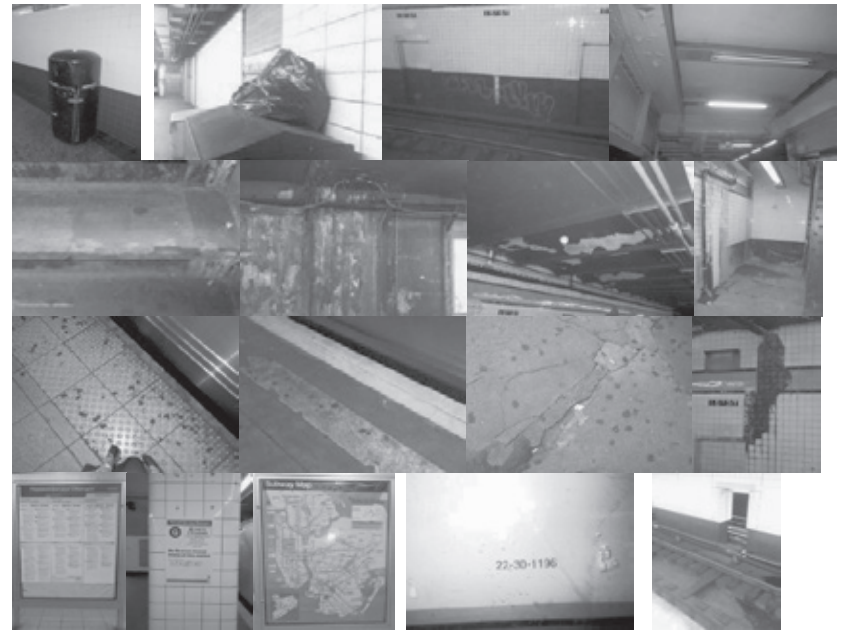
Picture Key by Question (from Left to Right) Row One: 1. Garbage Can; 3. Large Bag of Garbage; 5. Graffiti; 6. Broken Overhead Lighting. Row Two: 7. Crumbling Stair Edge; 8. Exposed Wiring; 9. Peeling Paint; 10. Water Damage. Row Three: 11. Proper Tactile Warning Strip; 11. No Tactile Strip; 12. Floor Cracks; 13. Missing Wall Tiles. Row Four: 14. Service Notices; 14. Service Notices on a Pillar; 16. Large-Scale Subway System Map; 17. Commodity Number; Two Track-Beds.
