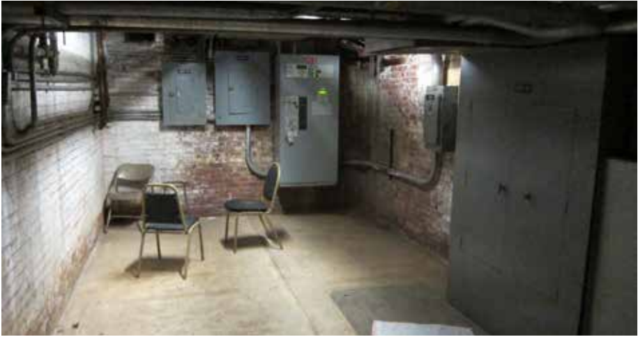
Emergency Lighting Panel, Emergency Power Panel & Automatic Transfer Switch in Basement.
