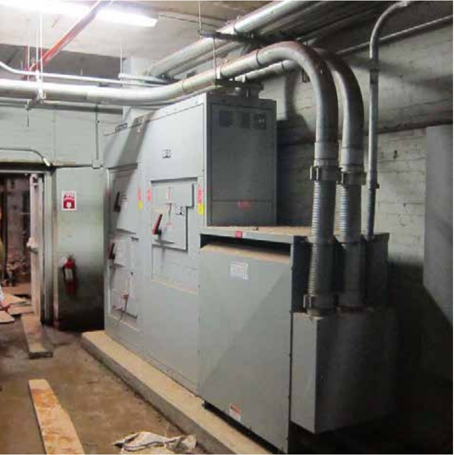
208V main switchgear and transformer in cellar level oB would need upgrade to match the 480V campus system.
