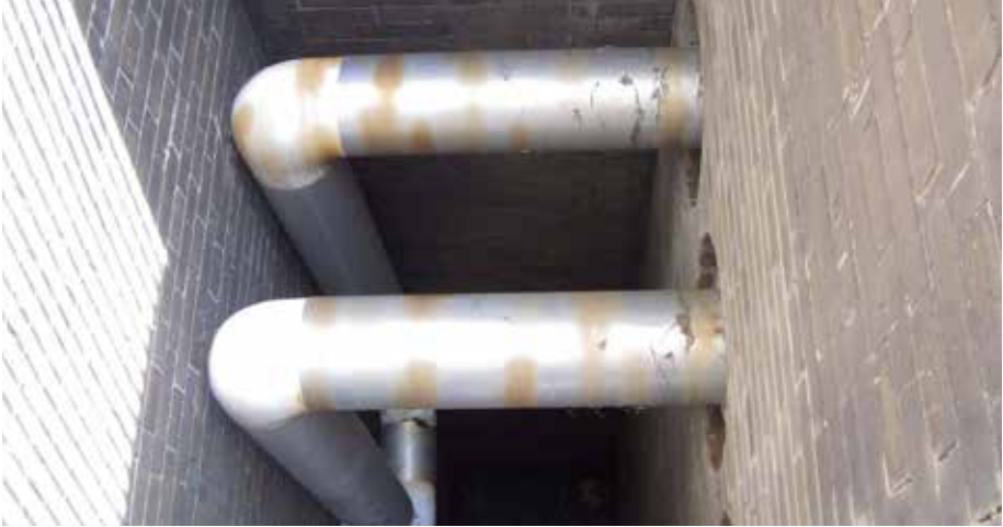
Campus steam main entering GML through SW areaway.
