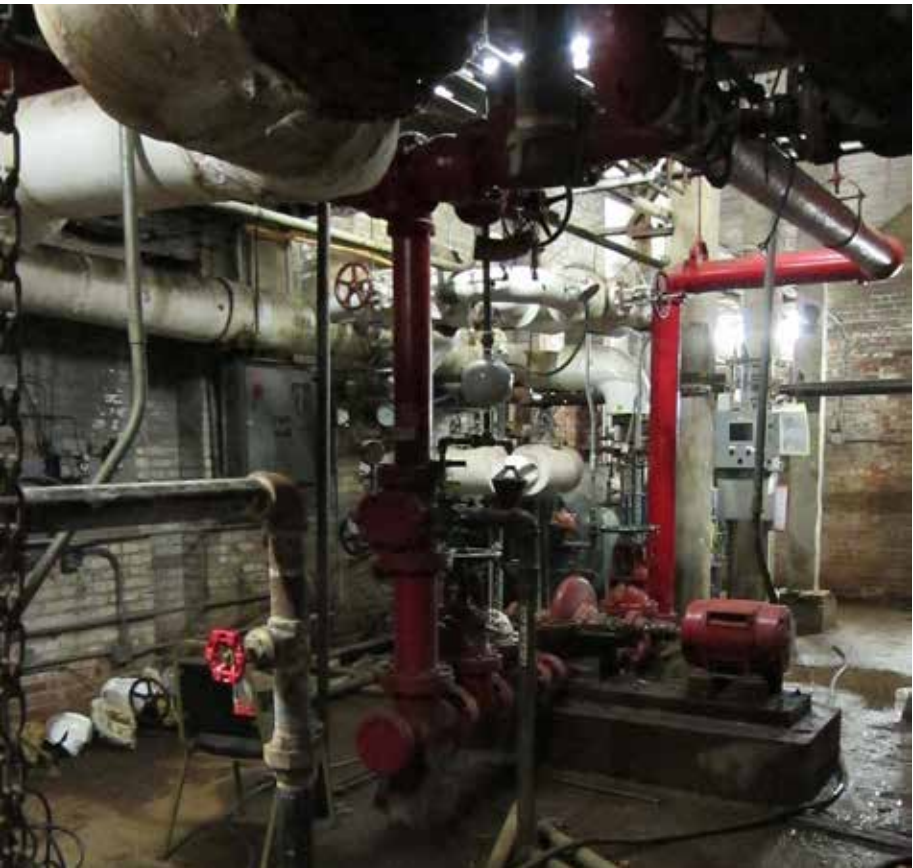
Space for services is ample in cellar level oB. The red sprinkler pump in the foreground at 208V, different than the campus system, and the steam generator behind is supplied by the network.
