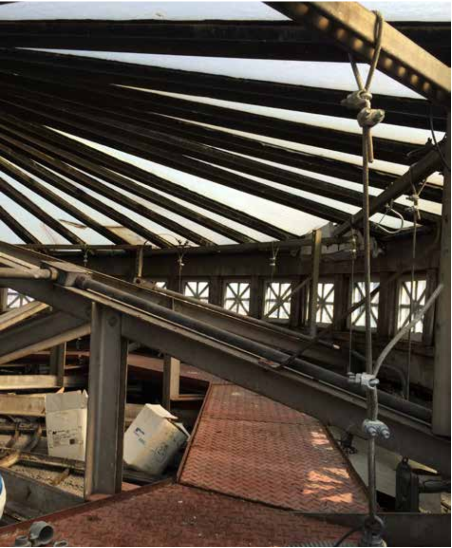
Project for the replacement of the cupola skylight awaits funding. New windows below the rafters would be operable to allow future smoke purge.
