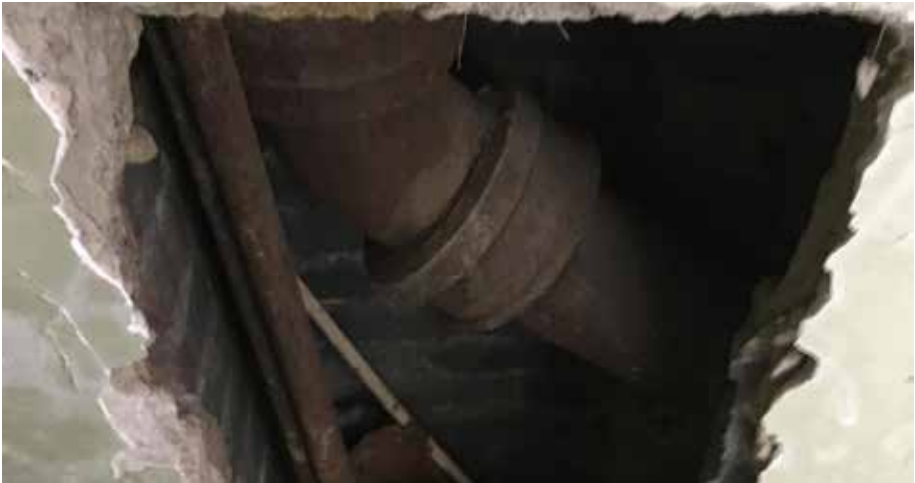
Existing stormwater drain exposed in Attic Level.
