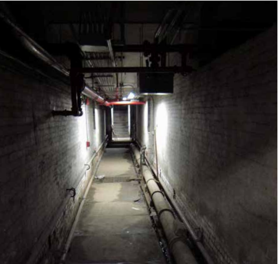
Combined sanitary / storm main runs north-south through the level oB cellar corridor, and sprinkler piping is suspended from the ceiling.
