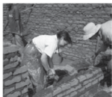
Building houses for Habitat for Humanity, Malawi
